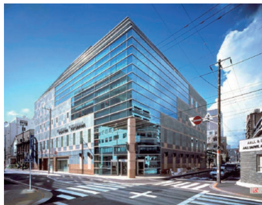
Workpia Yokohama Convention Facility, Yokohama, Japan.
